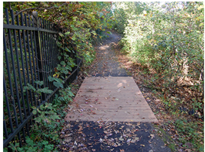
Above left: fixing the end of the boardwalk by raising the approach. Right: Smoothing the path by covering the water channel.
