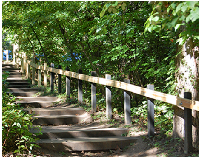
New handrail along the front steps replaces the original 1975 handrail.
