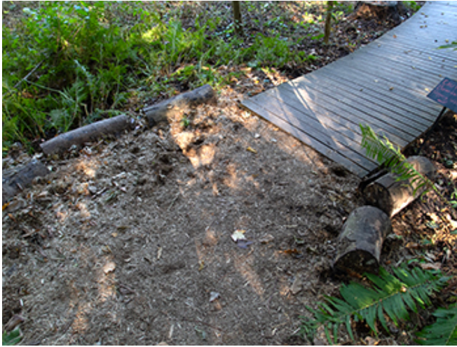
Above left: fixing the end of the boardwalk by raising the approach. Right: Smoothing the path by covering the water channel.
