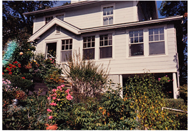
The steps and garden leading to the main floor entrance
